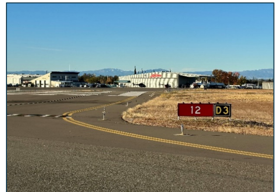
Airfield signage and taxiway lighting
